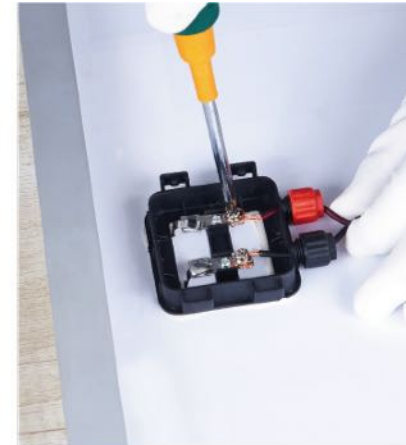
connect the cables with the solar panel
