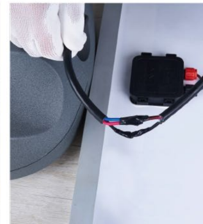
connect the lamp cables with the solar panel cables, installation finish
